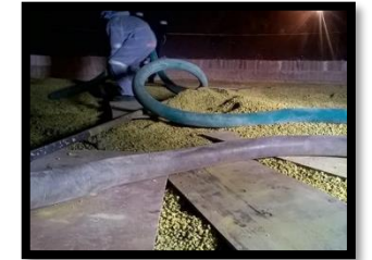
Inadequate Offline Catalyst Cleaning
